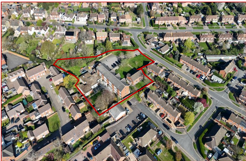
Rear / Side Elevation (South East)
